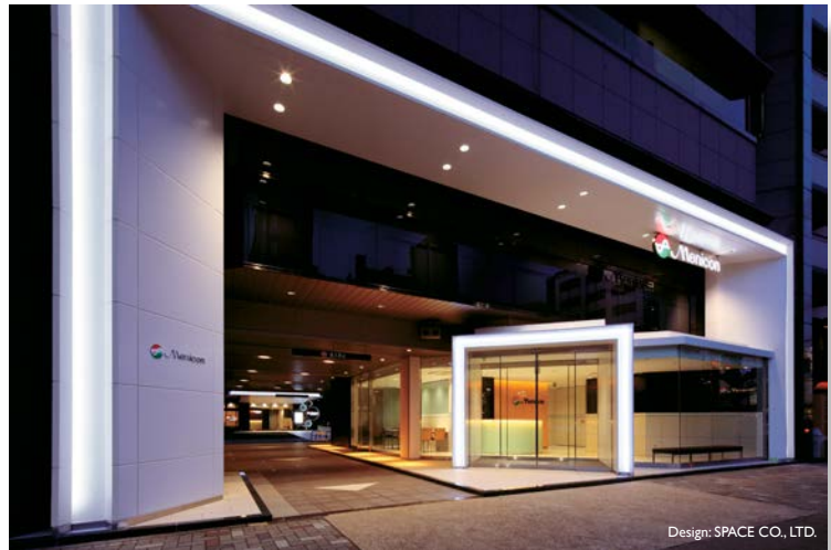
Indirect TokiLum 6500K highlights the entrance to this building.
